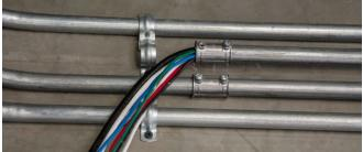
**NEC Chapter 9** is used for combinations of conductors of different sizes or insulation types installed in the same conduit or tubing.
